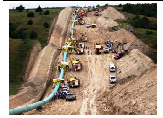
Figure 6.0.1 – Leveled work corridor for pipeline installation, showing cut hillsides and evident dewatering into the pipeline trench. Heavy equipment and pick-up trucks provide a scale.
