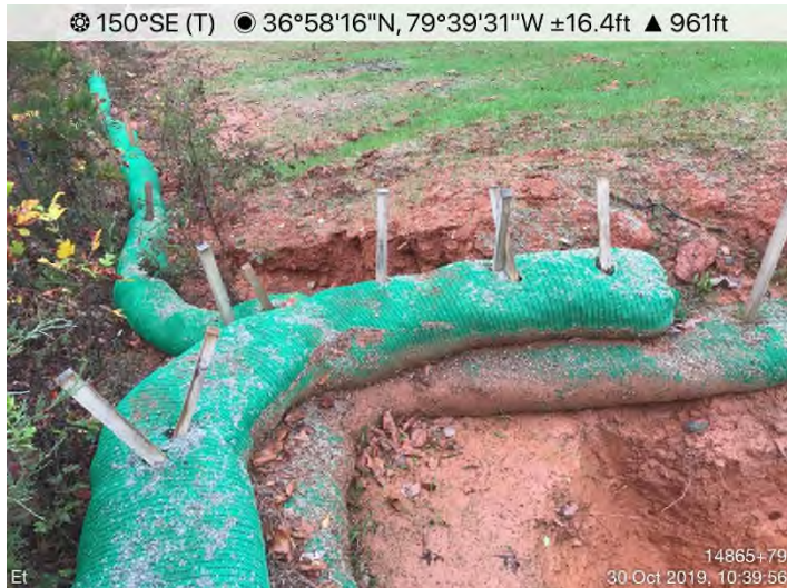
Fig. 3: STA 14867+00 – End-treatment bypassed. Maintenance needed.
