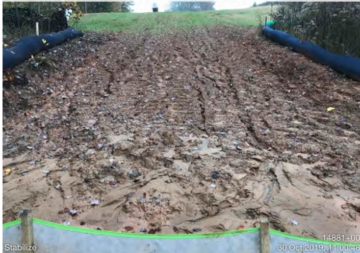
Fig. 9: STA 14881+00 – Stabilize slope/repair erosion adjacent to S-CD8.
