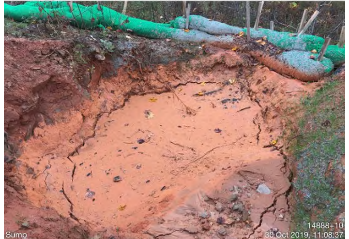
Fig. 12: STA 14888+10 – Sump maintenance needed.
