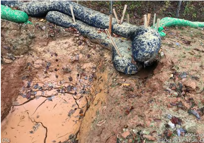
Fig. 19: STA 14904+00 – CFS undermined. Maintenance needed.
