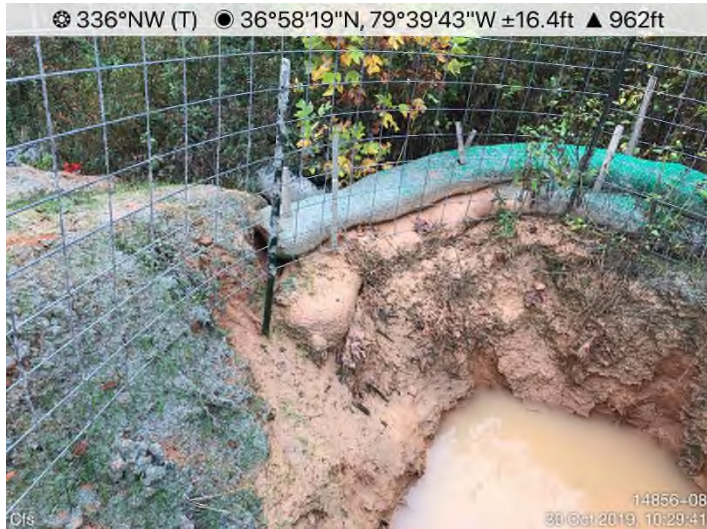
Fig. 3: STA 14867+00 – End-treatment bypassed. Maintenance needed.
