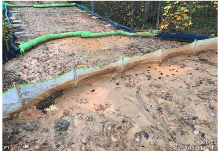
Fig. 12: STA 14888+10 – Sump maintenance needed.
