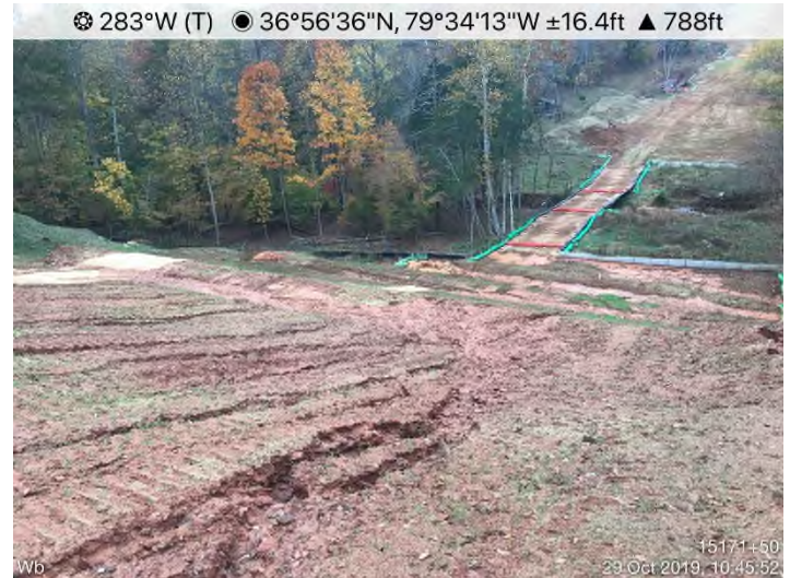
Fig. 4: STA 15169+58 – CFS overtopped. Maintenance needed.
