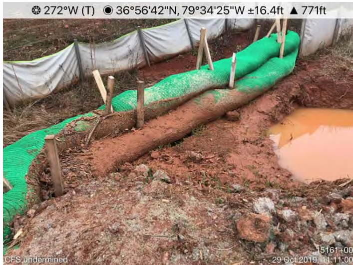
Fig. 9: STA 15161+00 – CFS undermined.
