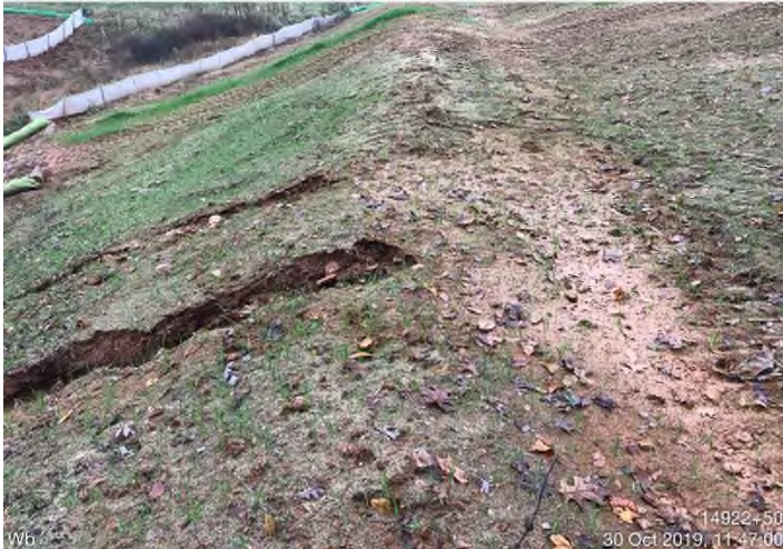
Fig. 23: STA 14922+50 – Waterbar maintenance needed.
