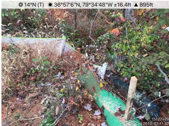
Fig. 19: STA 15126+00 – CFS undermined.
