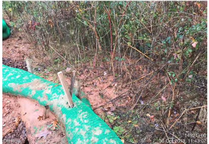
Fig. 24: STA 14922+50 – CFS undermined. Maintenance needed.
