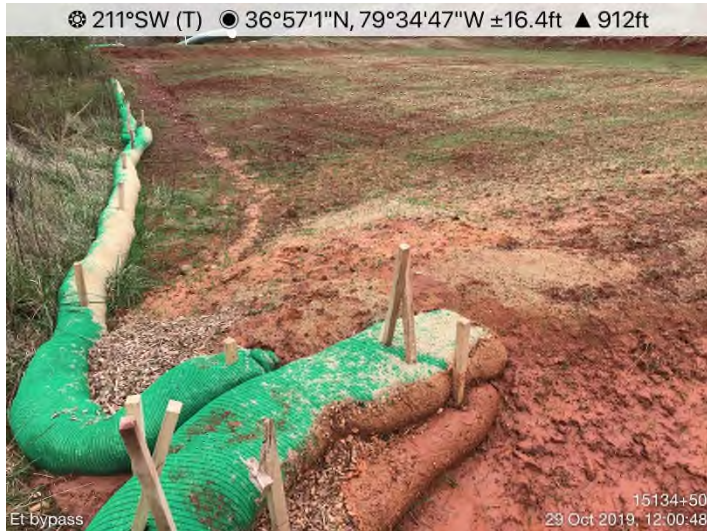
Fig. 15: STA 15128+65 – CFS undermined. Maintenance needed.
