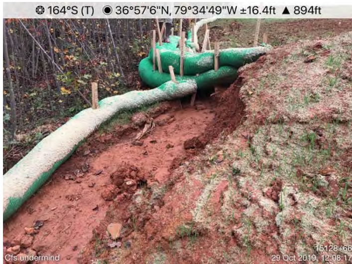
Fig. 15: STA 15128+65 – CFS undermined. Maintenance needed.
