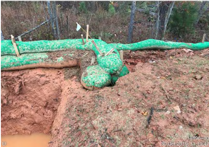
Fig. 19: STA 14904+00 – CFS undermined. Maintenance needed.
