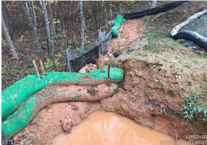
Fig. 11: STA 14882+00 – CFS undermined. End-treatment discharges onto ROW.
