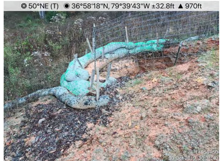
Fig. 4: STA 14869+60 – End-treatment undermined. Maintenance needed.
