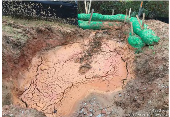
Fig. 8: STA 14880+00 – Sump maintenance needed.
