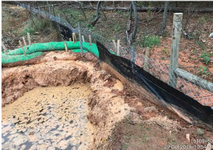
Fig. 7: STA 15162+25 – CFS maintenance needed.
