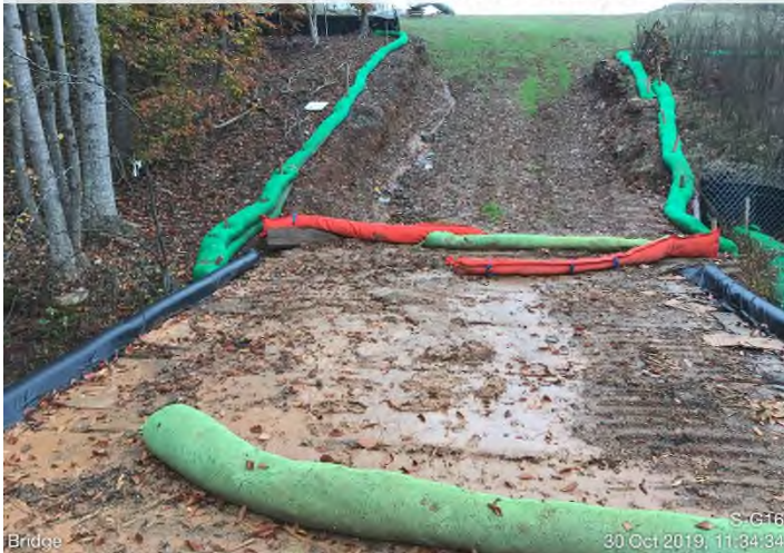
Fig. 21: STA 14916+26 – Clean sediment off bridge. Stabilize and repair slope adjacent to S-G16.
