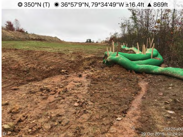
Fig. 21: STA 15125+00 – CFS end-treatment bypassed. Maintenance needed. Waterbar lower than CFS outlet.
