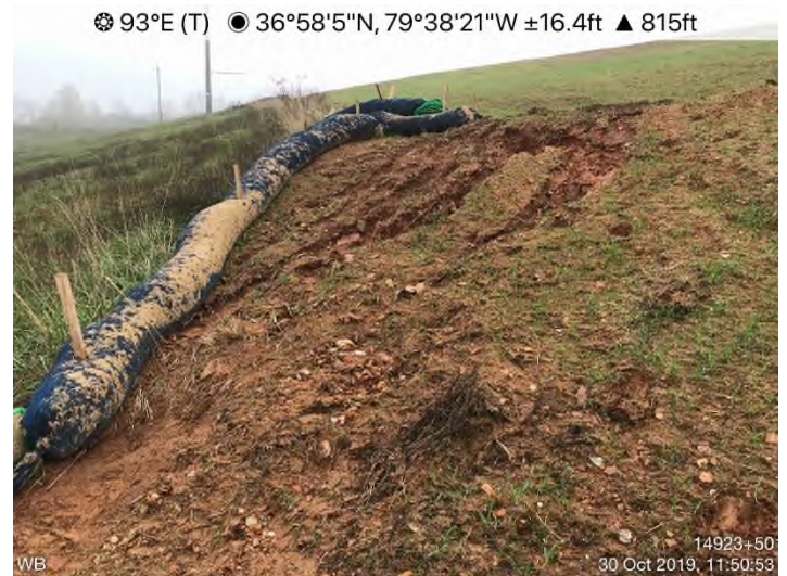
Fig. 26: STA 14923+50 – Waterbar maintenance needed.
