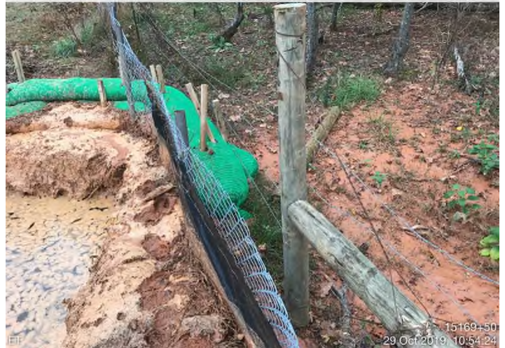
Fig. 8: STA 15162+00 – P1 undermined from channelized flow.
