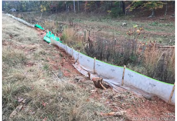
Fig. 8: STA 15162+00 – P1 undermined from channelized flow.
