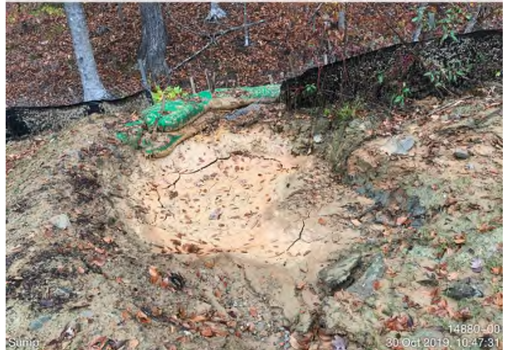
Fig. 8: STA 14880+00 – Sump maintenance needed.
