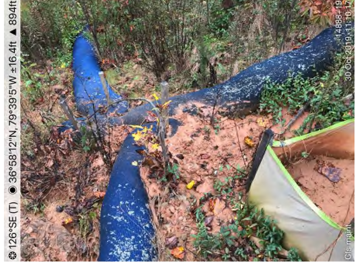
Fig. 16: STA 14888+75 – Stabilize slope/repair erosion adjacent to S-AB8.
