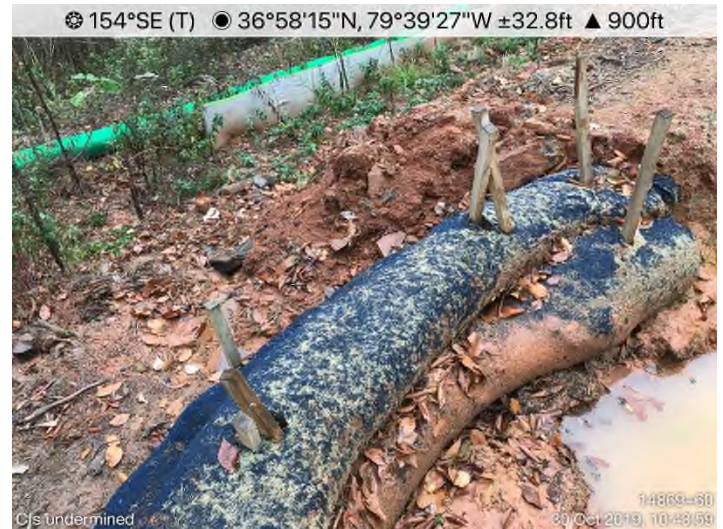
Fig. 4: STA 14869+60 – End-treatment undermined. Maintenance needed.
