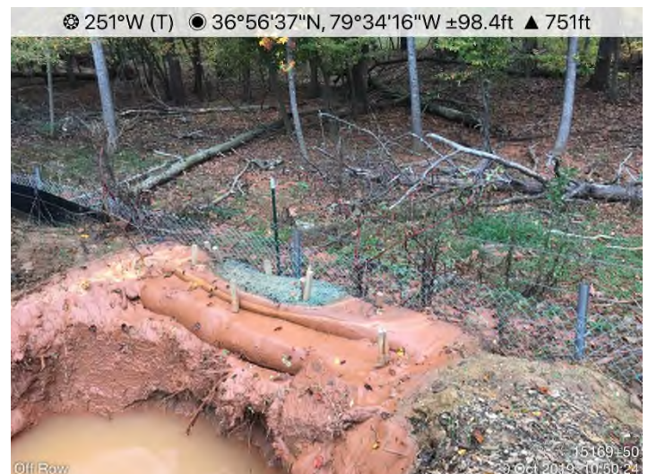
Fig. 4: STA 15169+58 – CFS overtopped. Maintenance needed.
