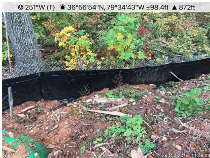
Fig. 11: STA 15142+00 – SSF undermined.
