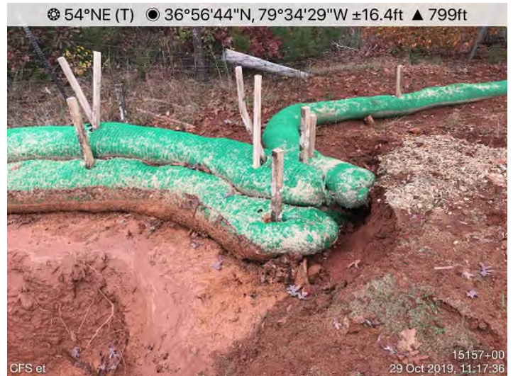
Fig. 10: STA 15157+00 – CFS end-treatment bypassed. Maintenance needed.
