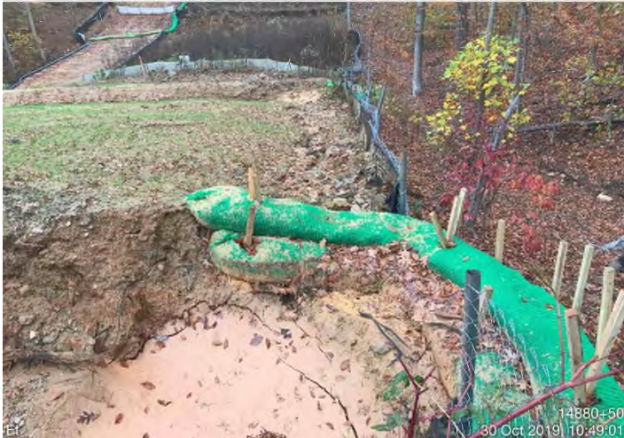
Fig. 7: STA 14872+50 – End-treatment discharges onto ROW. Maintenance needed.
