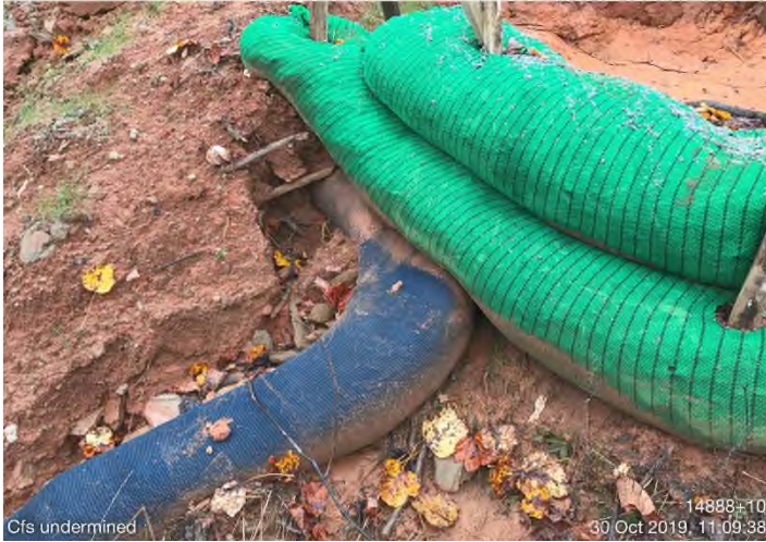
Fig. 15: STA 14888+60 – P1 maintenance needed.
