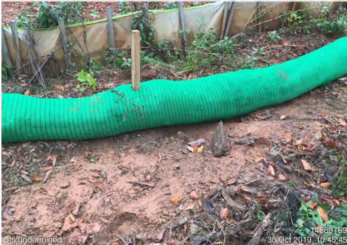
Fig. 7: STA 14872+50 – End-treatment discharges onto ROW. Maintenance needed.
