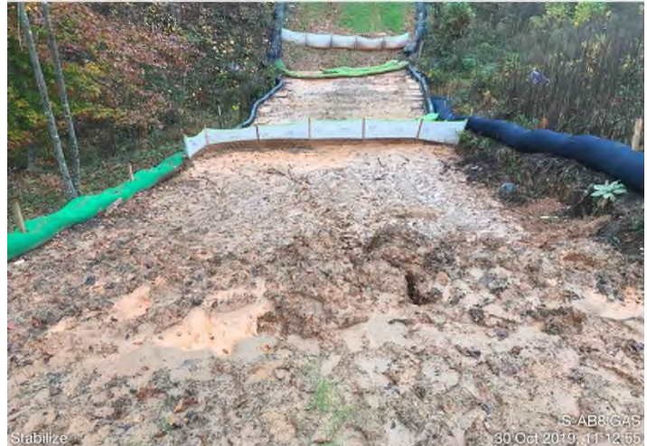
Fig. 16: STA 14888+75 – Stabilize slope/repair erosion adjacent to S-AB8.
