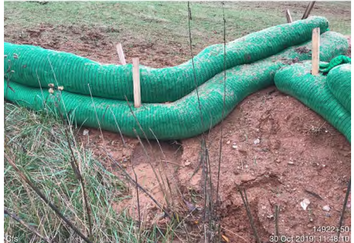
Fig. 24: STA 14922+50 – CFS undermined. Maintenance needed.
