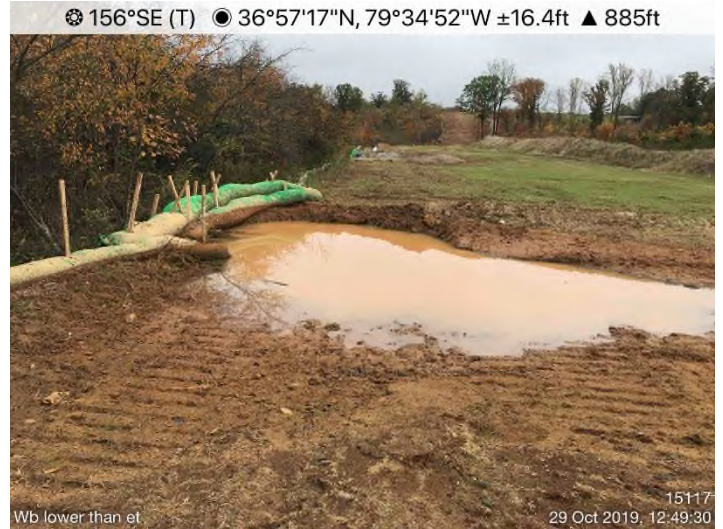
Fig. 22: STA 15117+00 – CFS end-treatment bypassed. Maintenance needed. Waterbar lower than CFS outlet.
