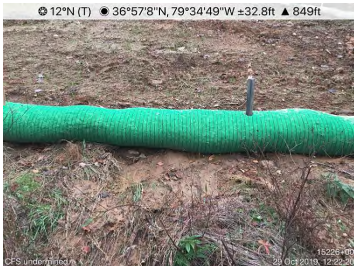
Fig. 19: STA 15126+00 – CFS undermined.
