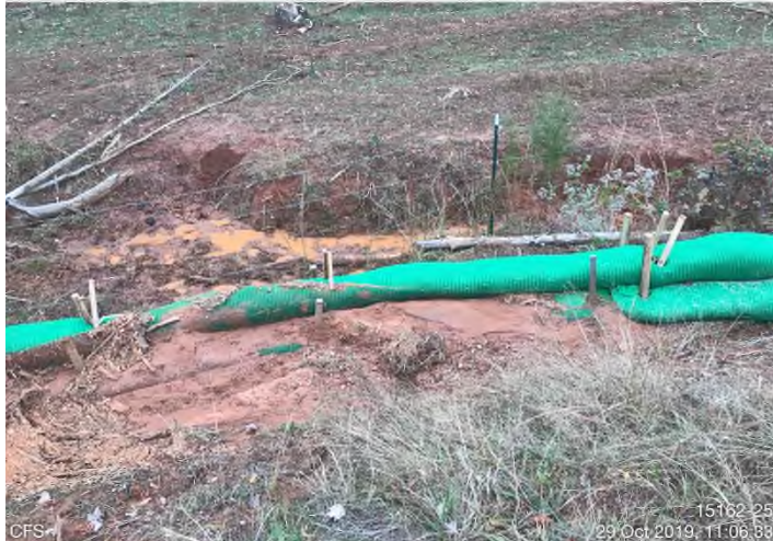
Fig. 7: STA 15162+25 – CFS maintenance needed.
