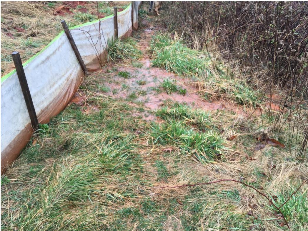
Figure 4 – Angle Property, February 23, 2019 (muddy water flowing under silt fence)
