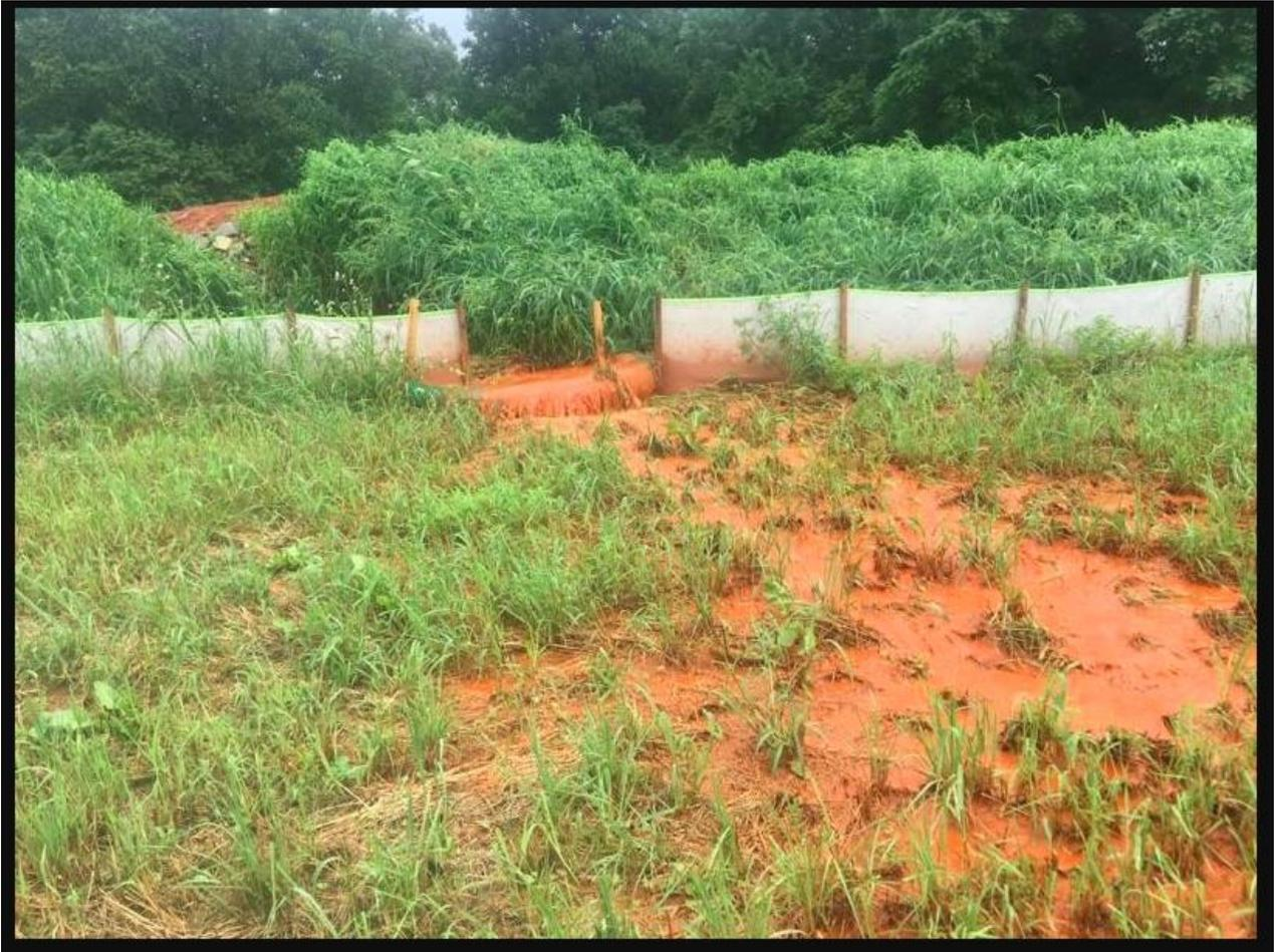
Figure 5 - Angle Property, August 3, 2018 (outlet from water bar failing)
